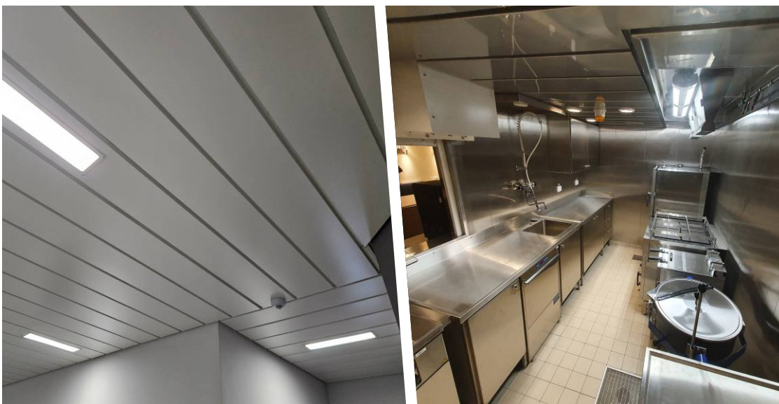
45-006 Self-Suspended sandwich construction B-0 and B-15 Class
